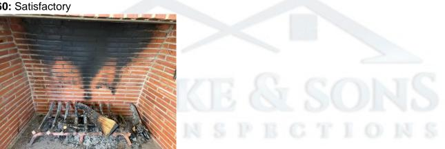
61: There are no glass doors installed. These could help minimize heat loss from the room when fireplace is not in use. When the fireplace is in use, they will eliminate embers from flying into the room and reduce the volume of room air sucked up the chimney.
