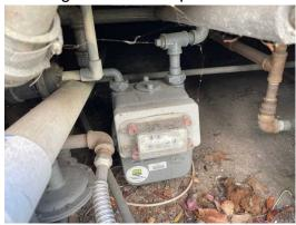
**190:** An automatic seismic gas shut off valve is not installed
