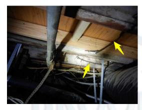
**s-257:** Attention needed: Unprotected electrical wires near attic access does not meet clearance requirements.
