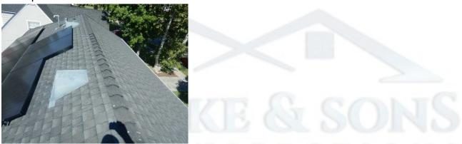
**67:** Fiberglass composition shingles. Fiberglass mat, asphalt impregnated. Shingles are applied in horizontal rows.
