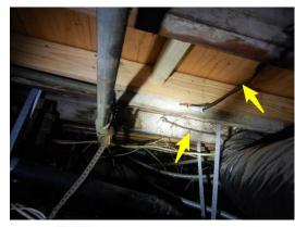
**257:** Attention needed: Unprotected electrical wires near attic access does not meet clearance requirements.
